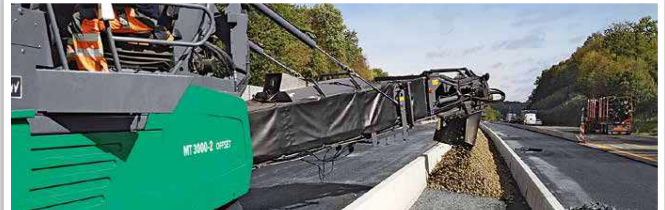
FILLING CAVITIES BETWEEN SAFETY BARRIERS
