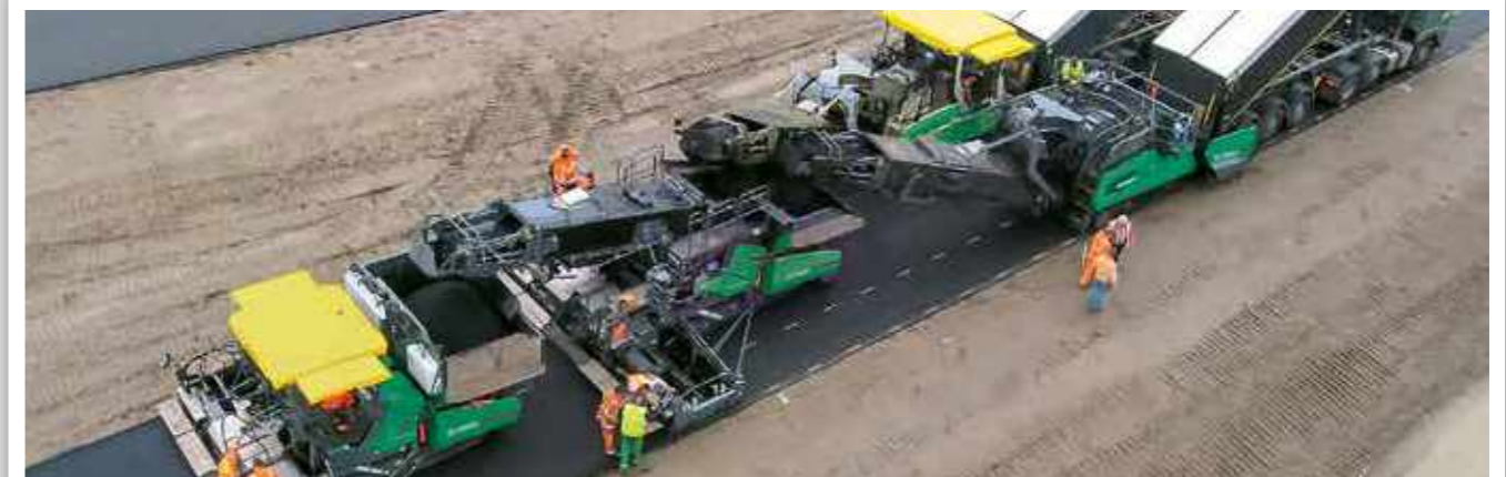
FEEDING PAVERS IN AN INLINE PAVE TRAIN
