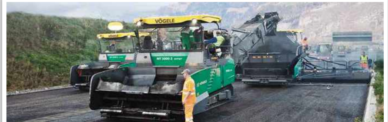
FEEDING PAVERS WHEN WORKING "HOT TO HOT"
